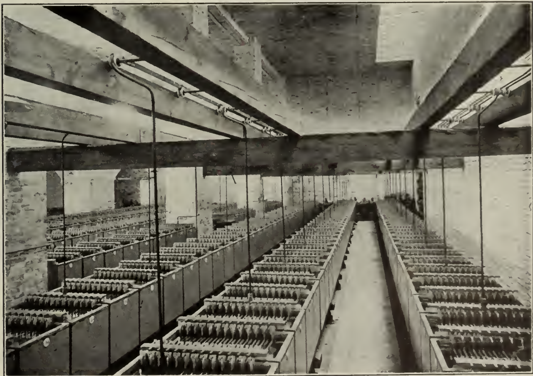
FIG. 5. ACCUMULATORS AT THE PORTA PIA STATION.
